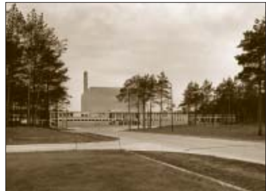
The BR1 building as completed in 1956
