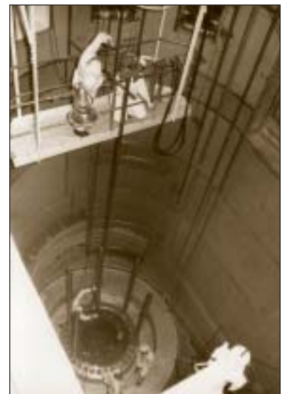
The introduction of nuclear fuel assemblies into BR3 in 1963
