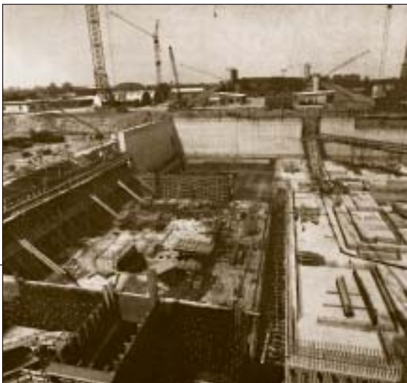
The SNR-300 in Kalkar during construction
